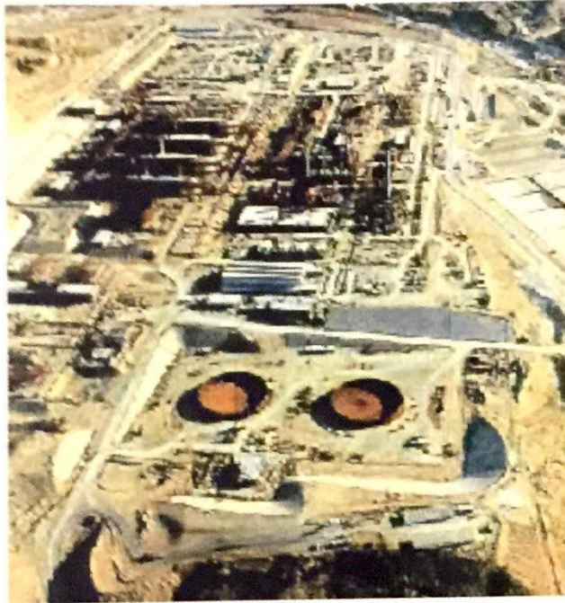
Figure 5 : Kargan Gas Processing Facility (courtesy of Nargan Company)
