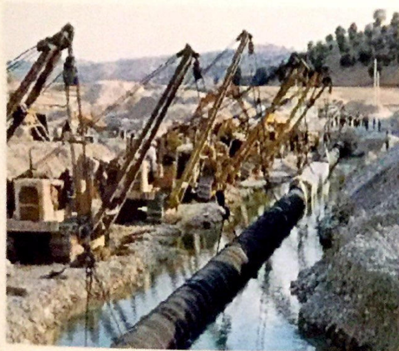
Figure 17: Pipelaying operation at river crossing (Courtesy of Tehran Jonoub)
