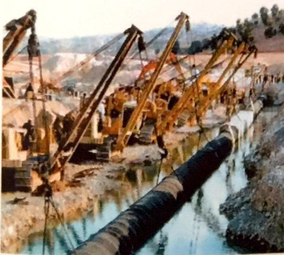
Figure 17 - Pipelaying operation at river crossing (Courtesy of Tehran Jonoub)
