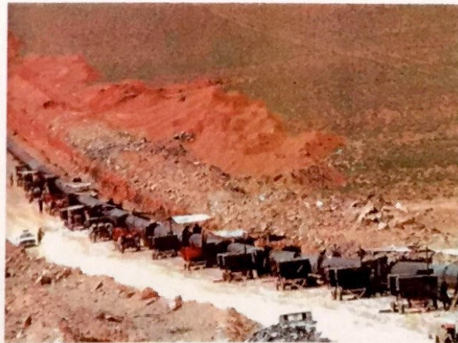
Figure 20 - 56" IGAT 2 Gas Trunkline (Courtesy of Tehran Jonoub)
